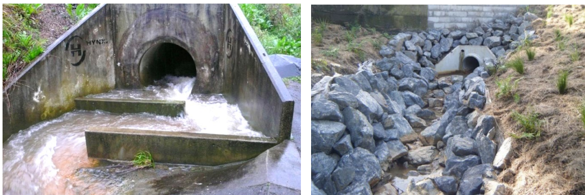
Figure 3-30: Left: Concrete apron and baffle blocks at outlet. Right: Rock riprap at outlet
