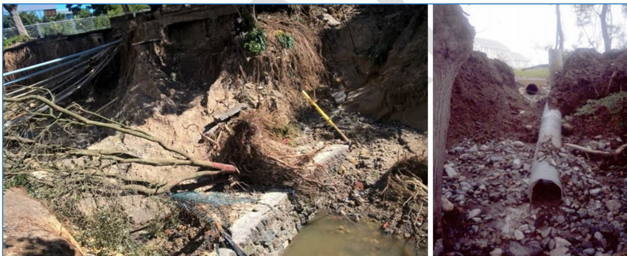
Figure 2-10: Culvert overtopping (outlet erosion after event) and pond failure due to piping pond failure. Photo courtesy of Stantec
