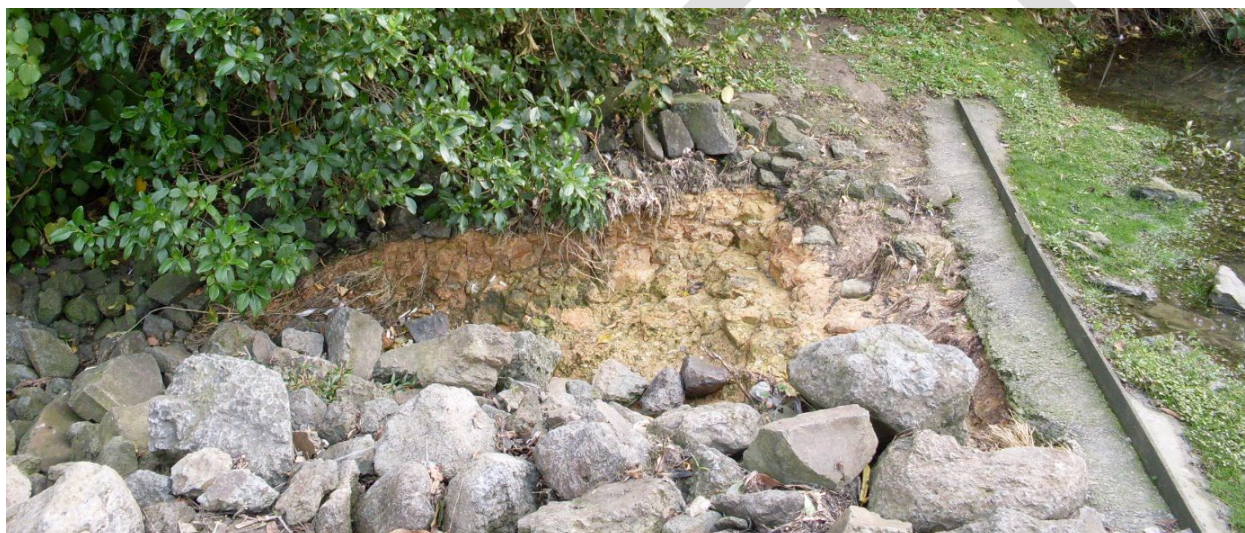
Figure 2-12: Outlet erosion of protected spillway downstream of pond level spreader
