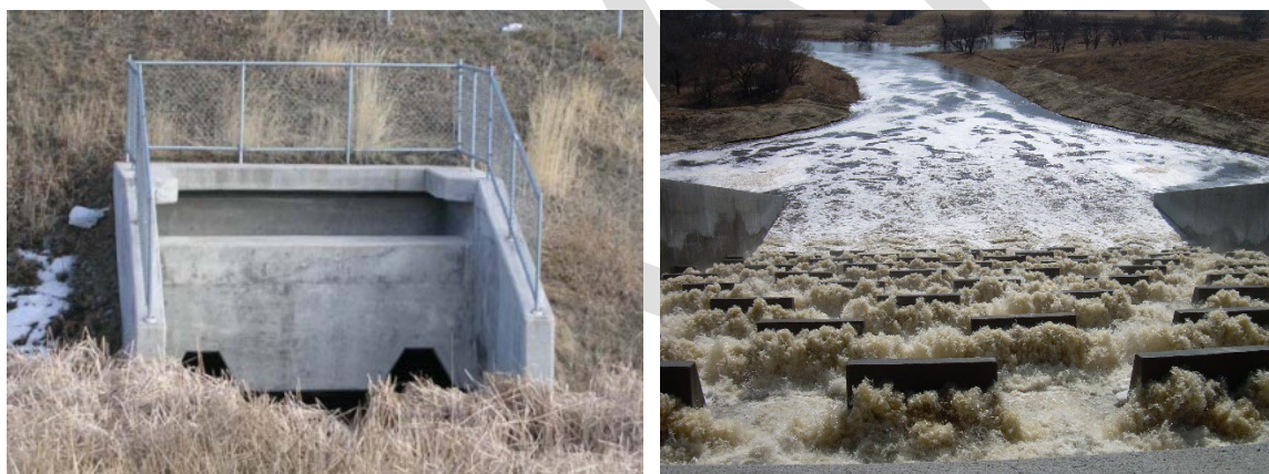
Figure 3-31: Left: Impact energy dissipater. Right: Baffled chute
