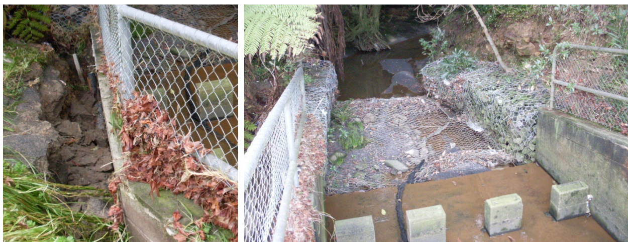
Figure 2-11: Left: Outlet erosion around structure (overland flow) Right: Erosion of riprap (excessive velocity and poor selection of Reno mattress fill rock)
