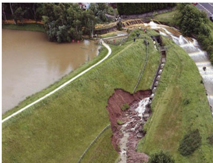
Figure 2-3: Erosion of dam and spillway and building foundations during large storms
