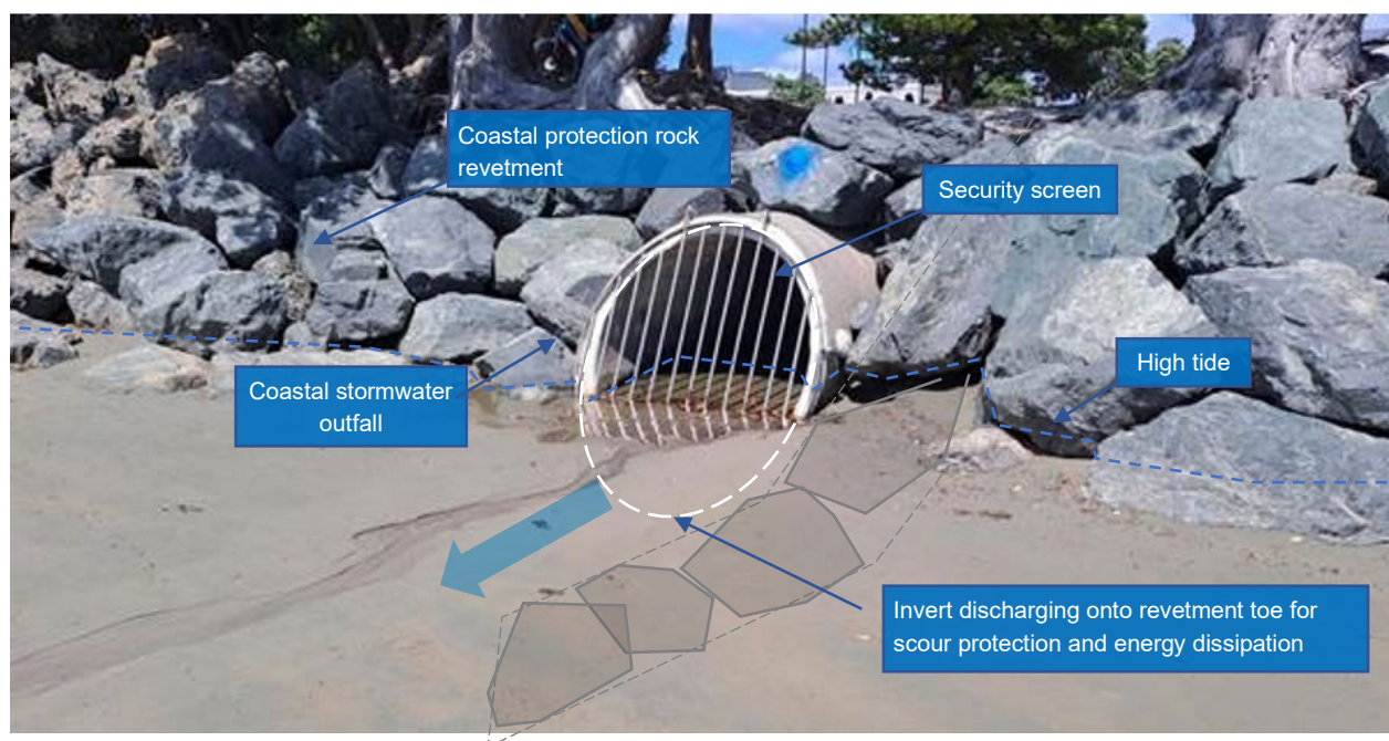
Figure 3-12: Example coastal outfall on the rear of a beach through rock revetment
