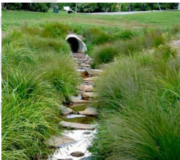
Figure 3-33: Rock riprap to protect outlet and stream channel
