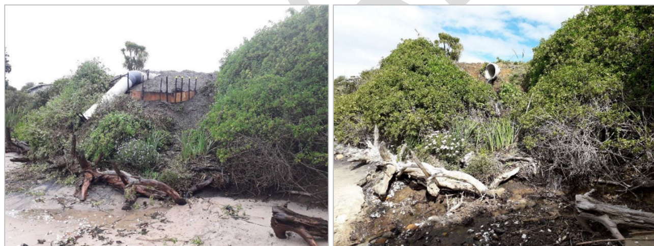
Figure 2-14: Left: Outfall suspended above beachhead, Right: Poor erosion control
