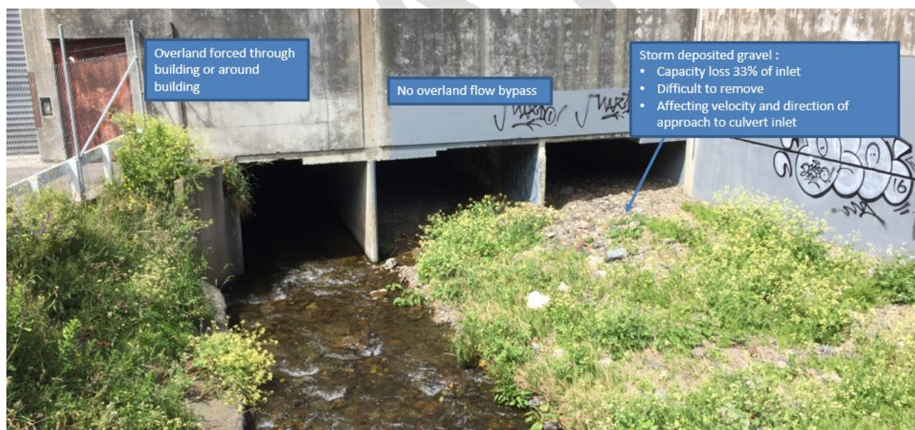
Figure 2-21: Sedimentation of a culvert inlet
