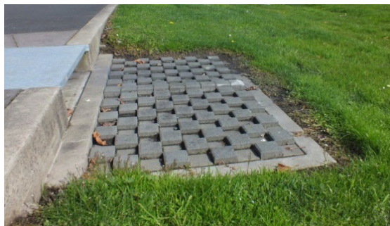
Figure 3-3: Level spreader outlet with energy dissipation onto grassed filter strip
