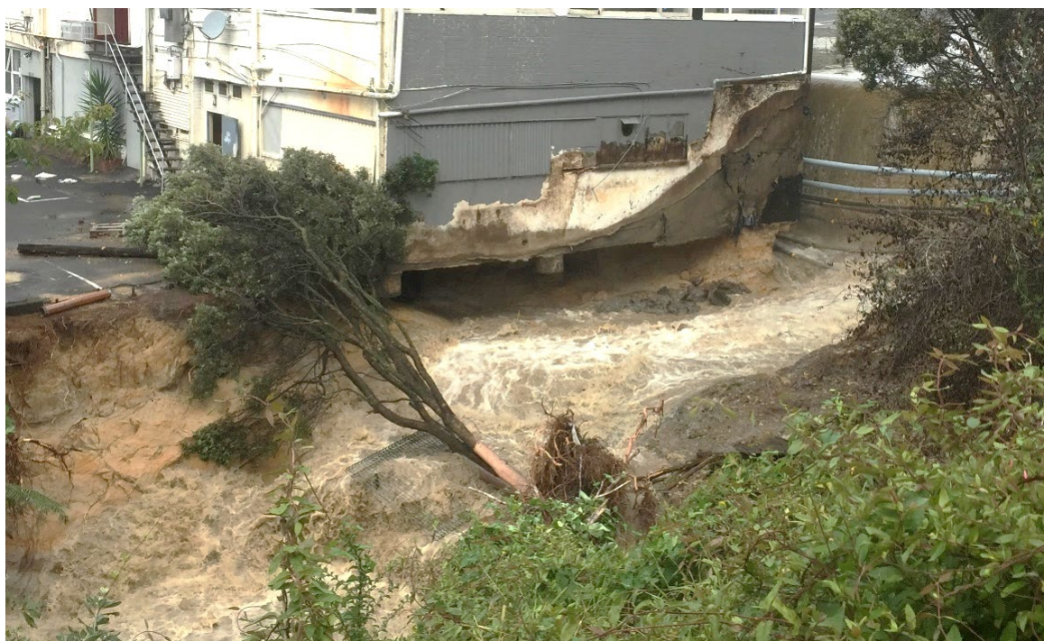
Figure 2-13: Overtopping led to excessive downstream erosion (outlet to downstream watercourse)
