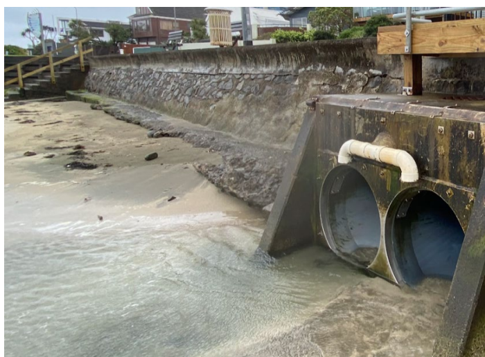
Figure 3-27: Inline check valve installed within a coastal outfall through seawall
