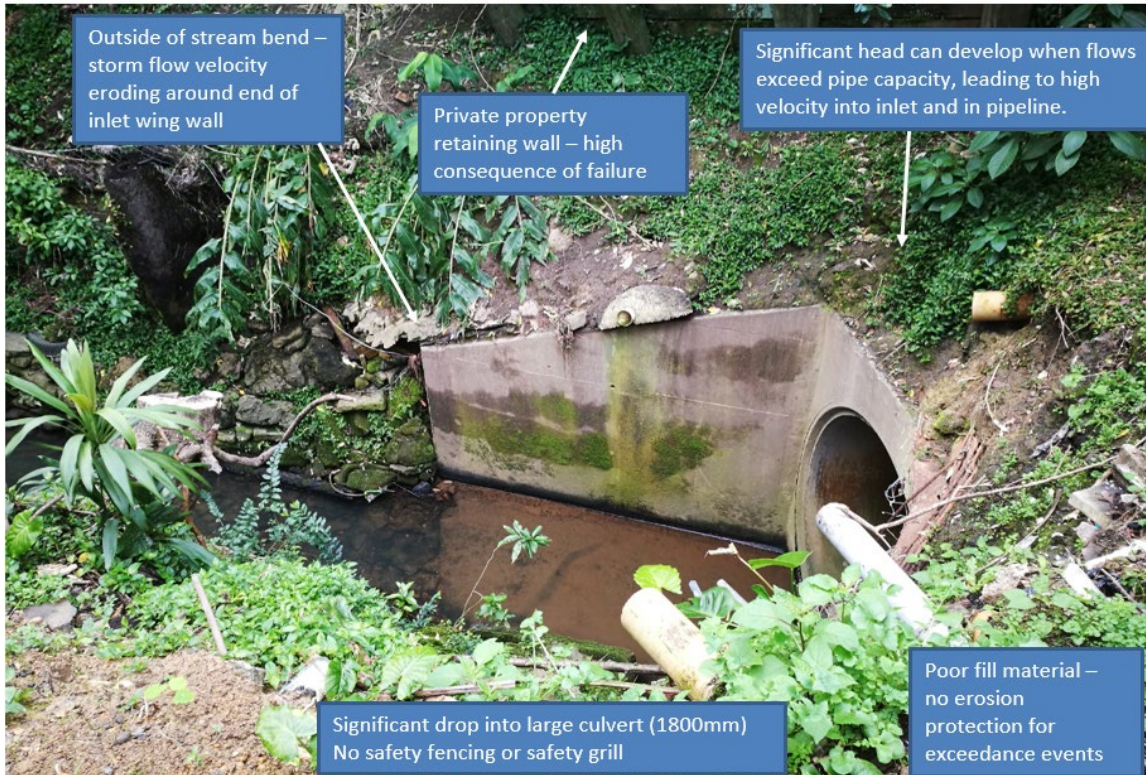
Figure 2-19: Velocity considerations for a culvert inlet
