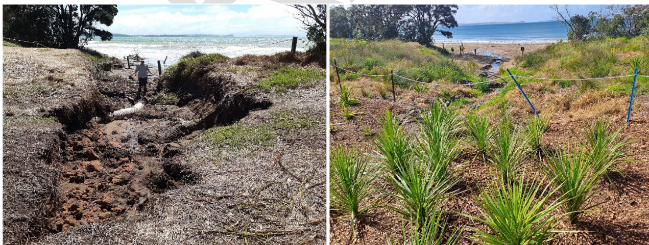
Figure 3-17: Left: Eroded coastal outfall structure
