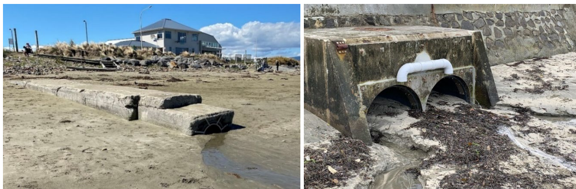
Figure 3-29: Examples of outfalls with sedimentation issues
