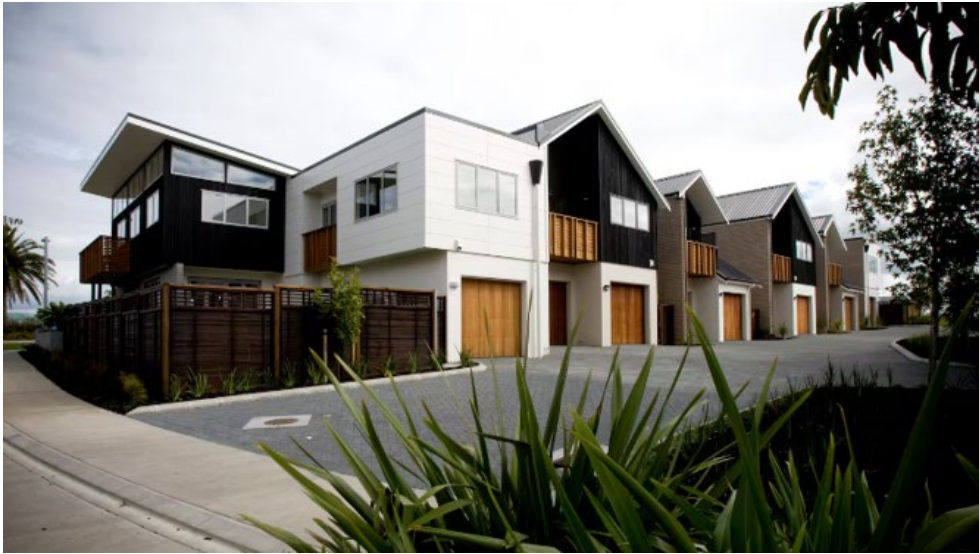
The dwellings have been designed with the rear of the units, including car access and garages facing a rear access lane. Main living spaces and dwelling fronts enjoy views and sun. Image credit: Dean Purcell for NZ Herald
