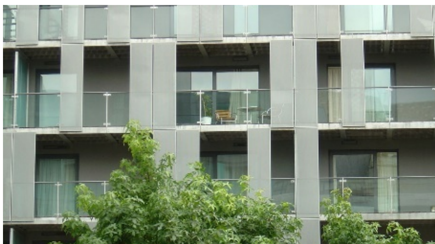
Thin mesh screens are used as part of the overall building design and provide privacy to each balcony. Balconies are integrated into the building to provide privacy for adjoining residents.
