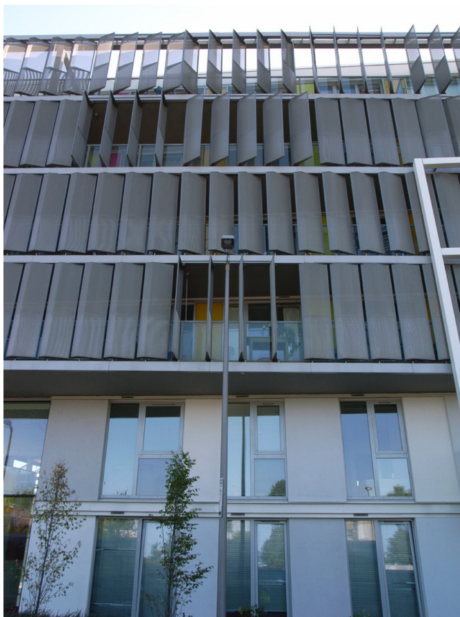
Rotating vertical louvers allow residents to modify and reduce passive solar gain.
