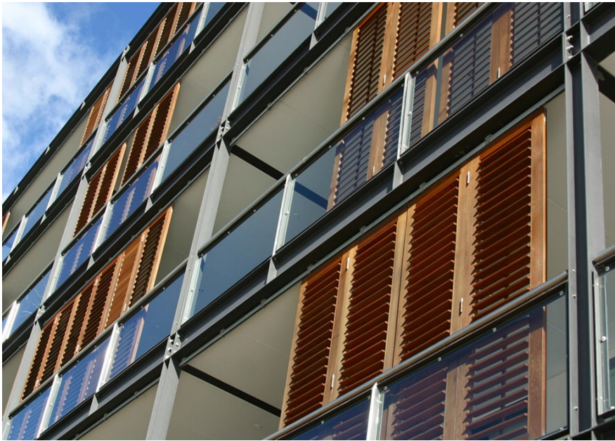
All the building elements the balcony structure, the balustrade, the wooden louvres are coordinated and carefully detailed.
