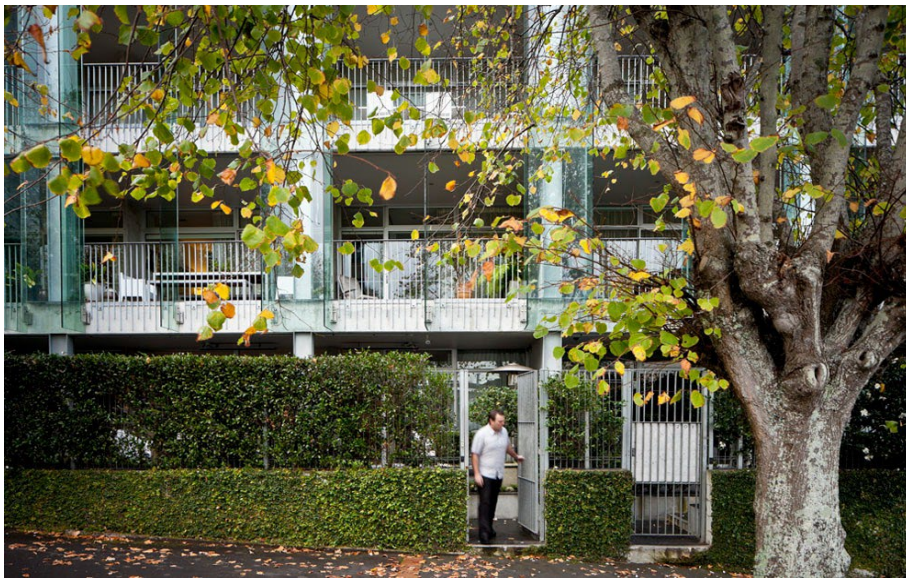
Planting provides privacy for ground floor dwellings.
