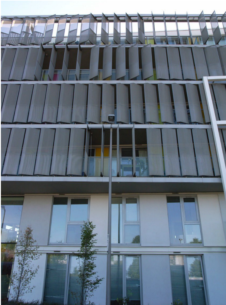
Rotating vertical louvres allow residents to modify and reduce passive solar gain.
