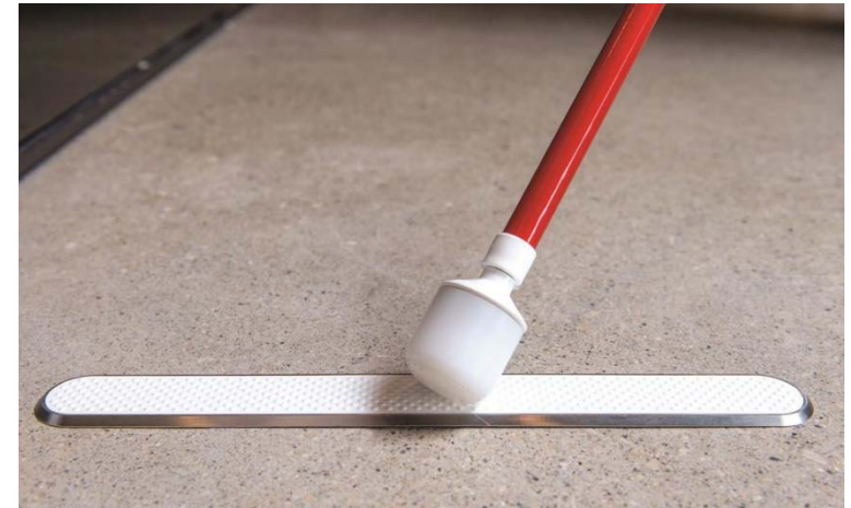
Cane detectable tactile strip (Sourced from CMHR, Ian McCausland).
