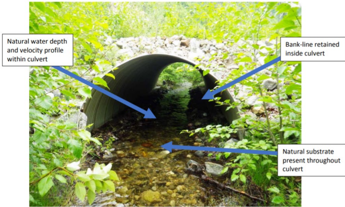
Figure 2 – An example of a stream simulation culvert design (Sourced from NZ Fish Passage Guidelines )
